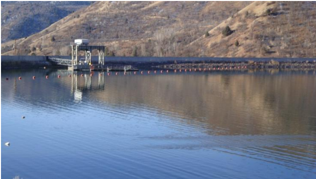
Oneida Narrows Dam (Danny White)
