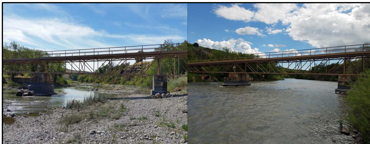
Figure 8: Comparison of water levels below Cutler Dam
