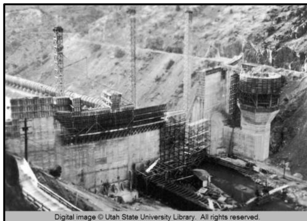
Figure 22: Construction of Cutler Dam, 1925. Image courtesy of USU Digital Archives
